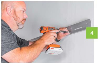
Secure French Cleat to desired location with correct mounting hardware.
