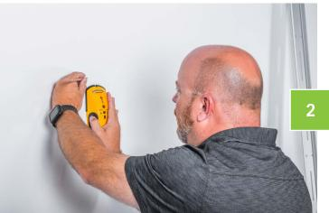
Locate metal or wood stud locations on wall for mounting.
