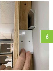
Attach safety locking plate to left or right side of mywall panels. This can be done as each panel is attached onto the wall.
