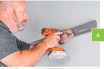
Secure French Cleat to desired location with correct mounting hardware. (not supplied)
