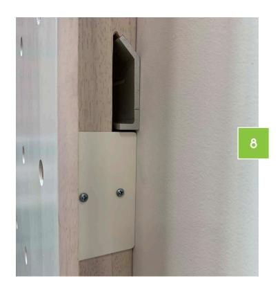
Attach safety locking plate to left or right side of mywall panel.
