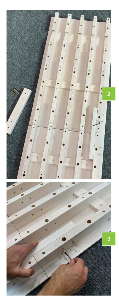
Lay myWall panels face down on a clean floor. Place both top and bottom sections next to each other. Top section has the cut-outs for the french cleat mounting at the top. The bottom panel has a lower open section at the bottom.
